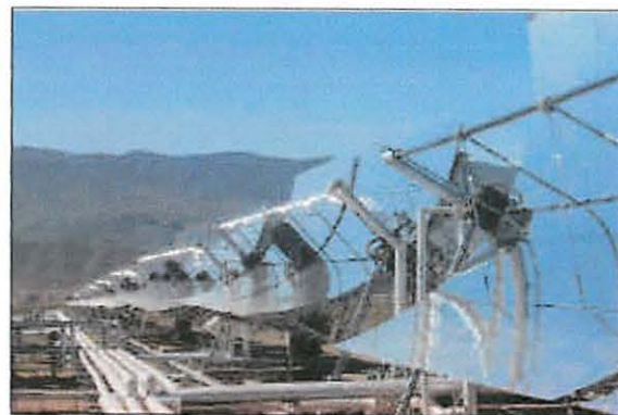
Direct steam generating parabolic trough test facility at the Plataforma Solar, Almeria, Spain
