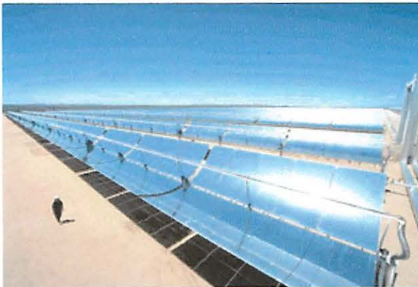
Parabolic trough system [Courtesy of SunLabs - Department of Energy]
