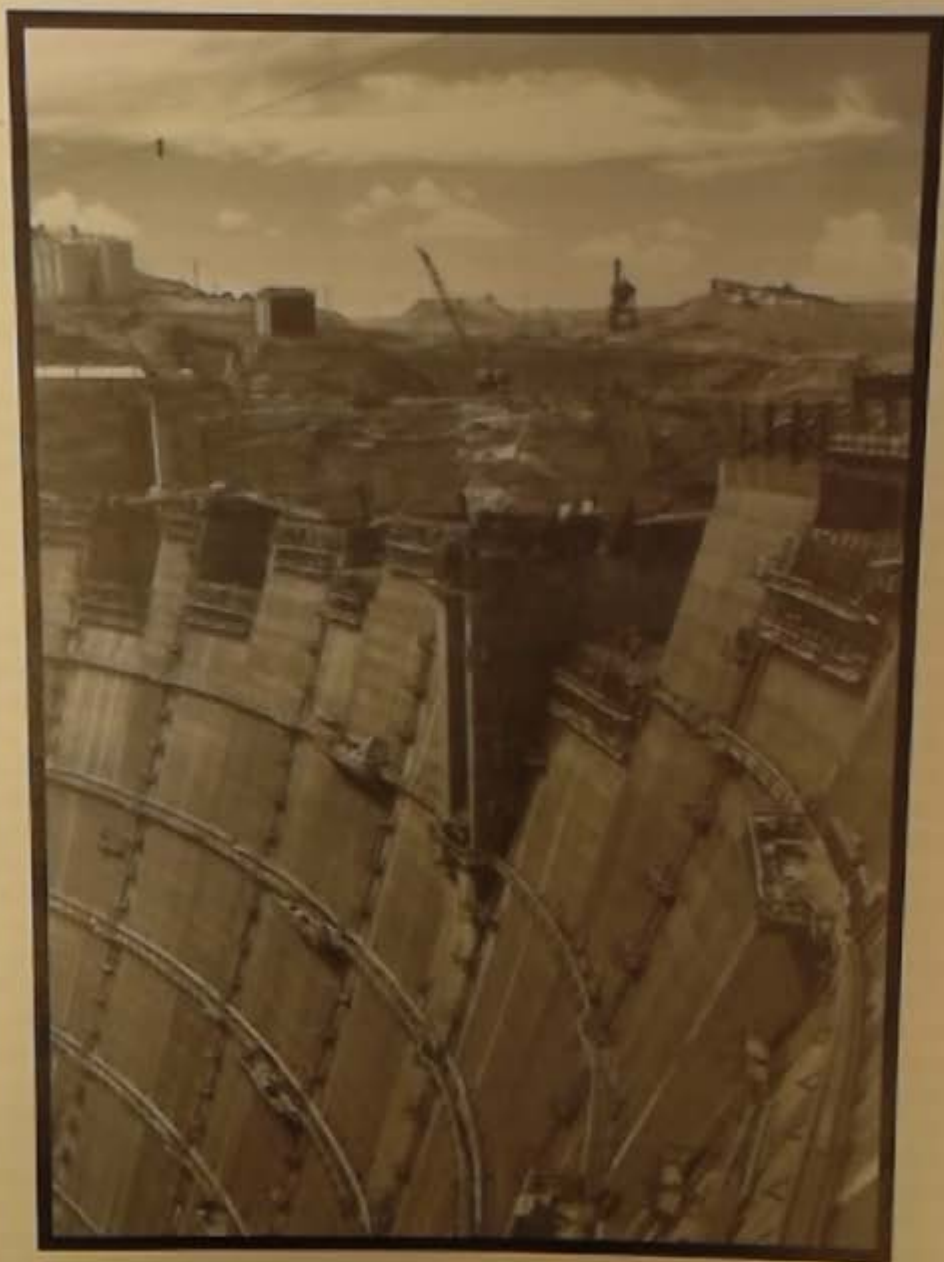
Glen Canyon Under Construction Colorado River Storage Project - April 9, 1965 Photographer - unknown
