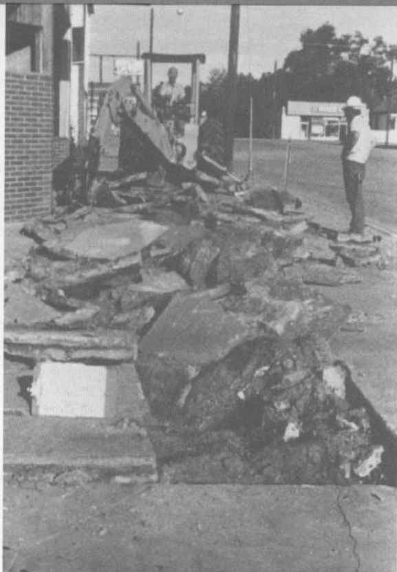
Vicinity Property Cleanup in Progress
