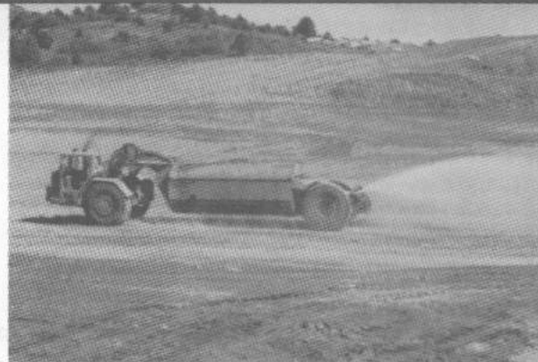
Dust suppression techniques are used during remedial action.
