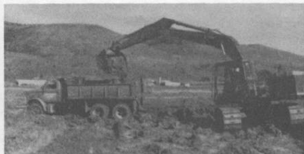
Remedial Action in Progress
