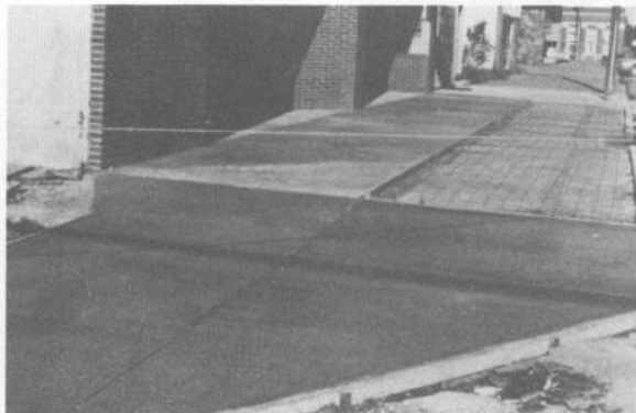
Restoration Following Tailings Removal
