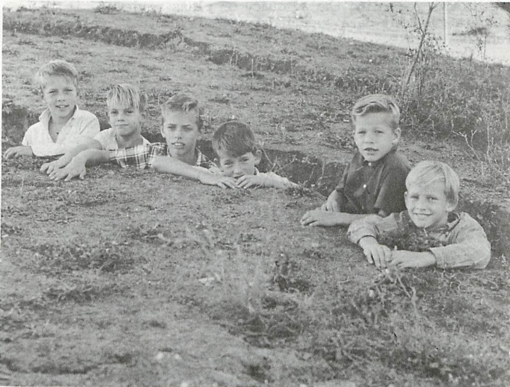
This soil has severe limitations for a building site. SCS PHOTO 3-7379
