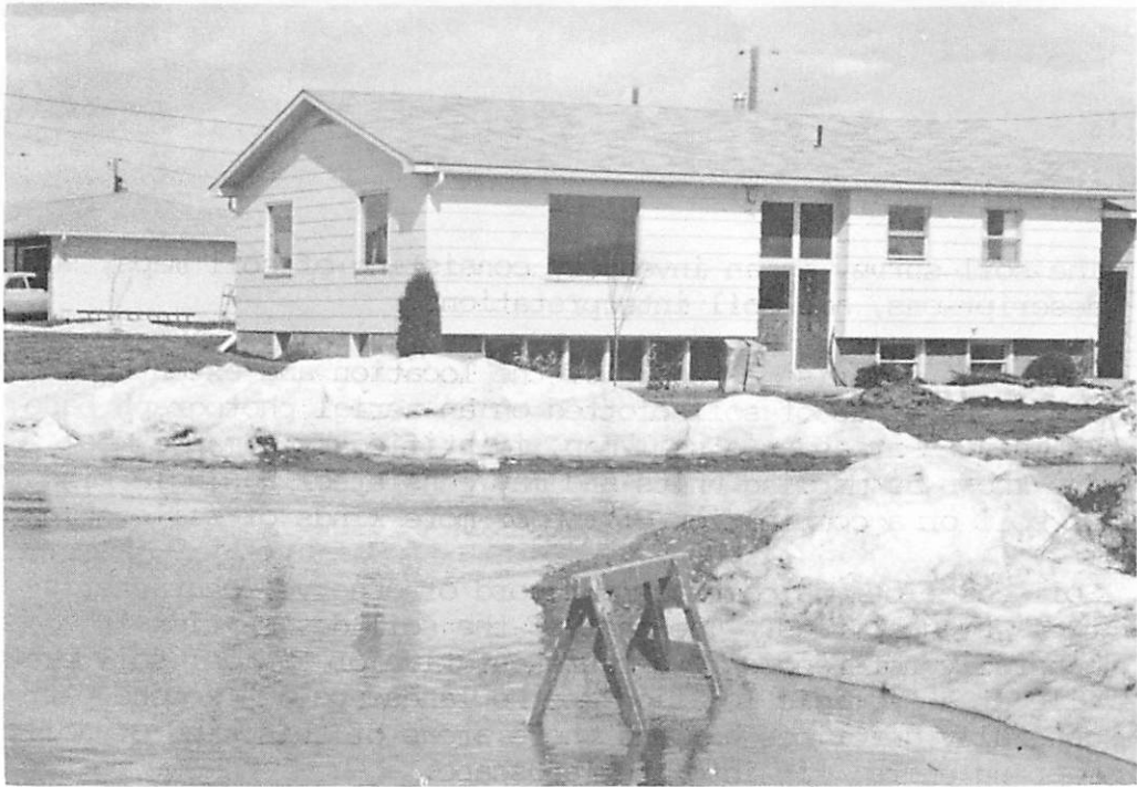
An inadequate drainage system causes problems. SCS PHOTO 11-P-490-3
