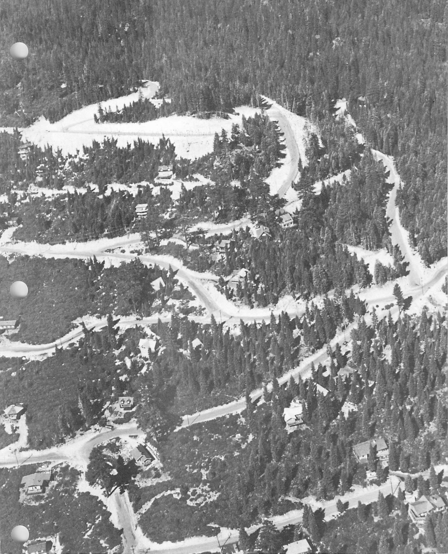
A subdivision site with severe slope limitations. SCS PHOTO 6-1173-15
