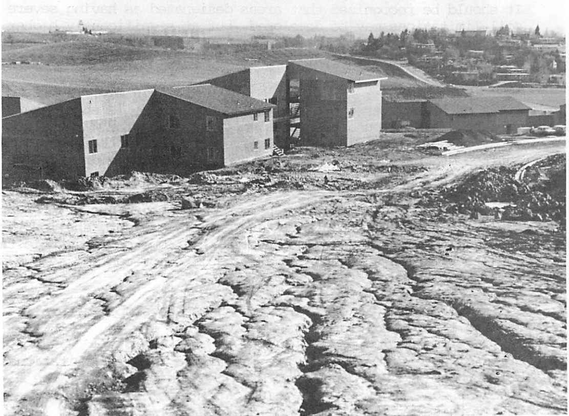
This site needs temporary protection such as mulch or vegetation.
