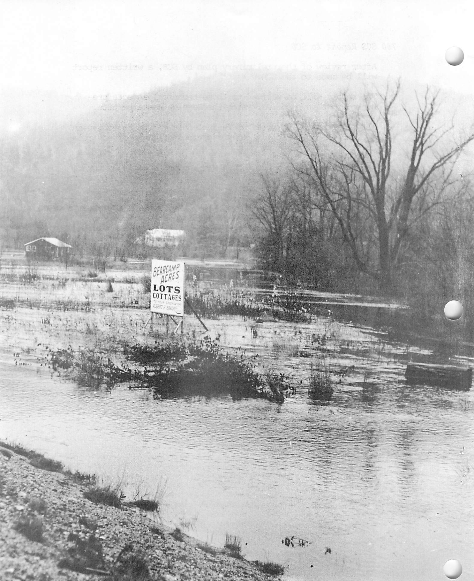
Floodplains make poor homesites. SCS PHOTO N. H. 171
