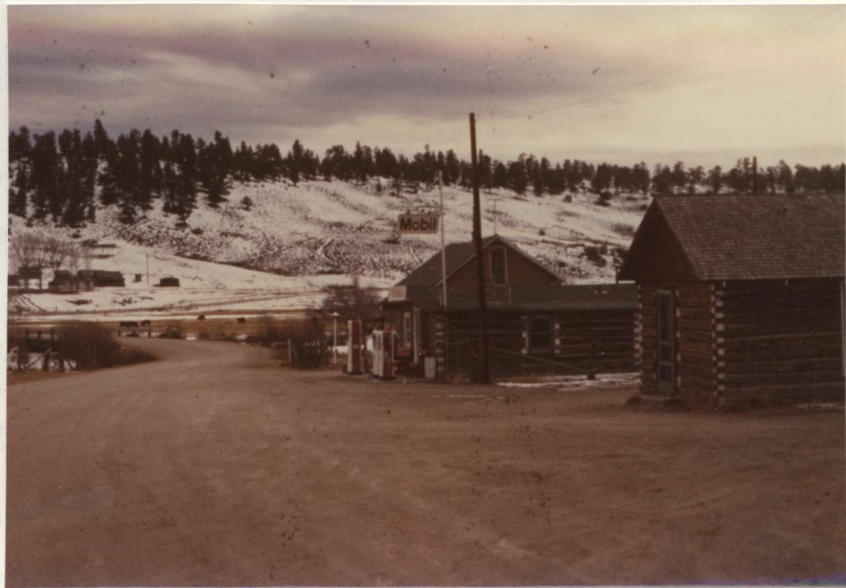
Fig. 6-8. Powderhorn Store. A local landmark behind which Fred Youman operated a weather station in the 1960's and where Station 8 is currently located.
