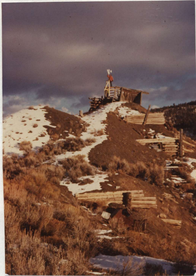
Fig. 6-5. Station 4. MRI and fenced shelter. Proposed location of tailings dam.
